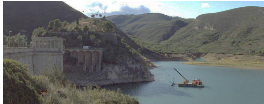
Works in Loriguilla Dam, www.chj.es
